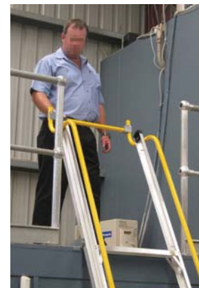
Safety access bar which flips over for access
